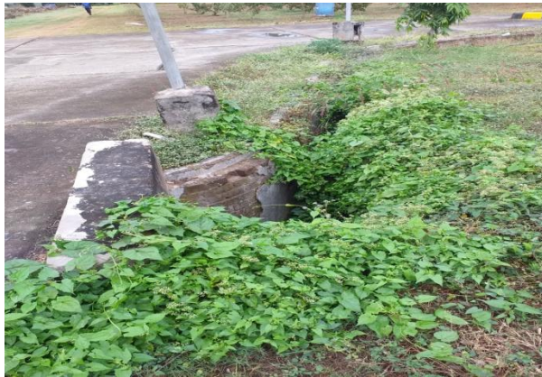
Before cleanliness drive
