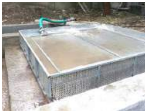
Fig. 2. On-line screen gravel filter functioning with layer of sand filter
