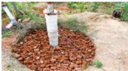
Fourth layer of brick flakes
