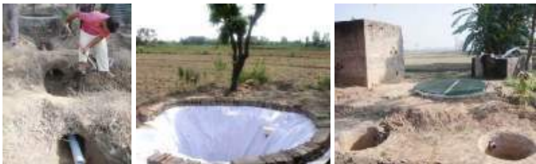
Fig. 1. Construction and lining of desilting pit
