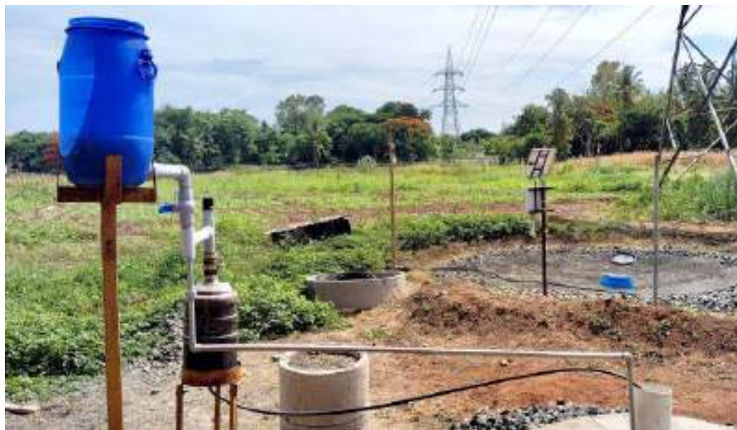
Fig. 3. View of field installation of sediment filter for groundwater recharge
