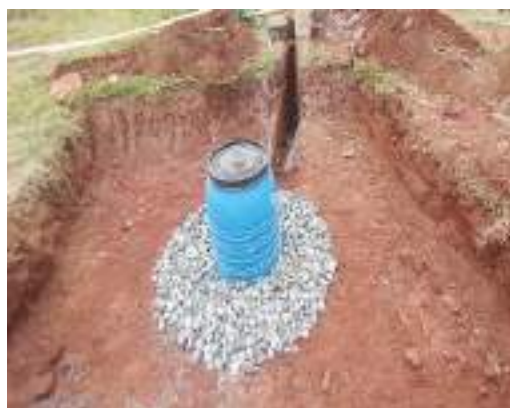
Fig. 4. Filling of 20-40 mm crushed stones around the central tank
