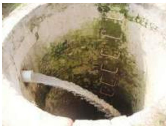
Fig. 2. Covering of abandoned well and entry of water into the well for recharge
