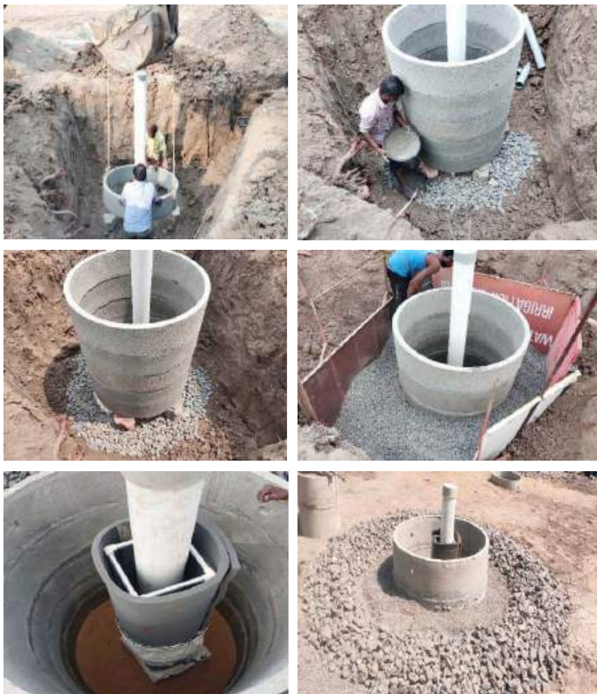
Fig. 2. Construction sequences of vertical flow sediment filter
