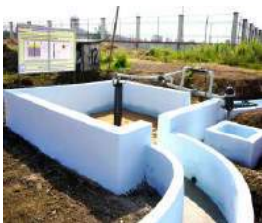
Fig. 3. Constructed recharge structure in IGKV research farm
