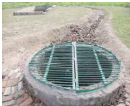
Fig. 2. Covering of abandoned well and entry of water into the well for recharge
