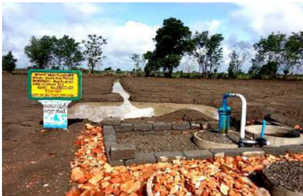
Fig. 2. Visit of farmers/trainees to groundwater recharge structure site
