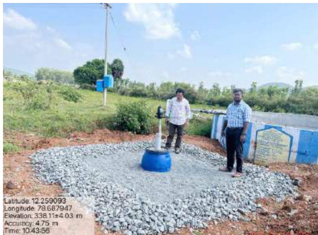
Fig. 5. Installation of horizontal flow sediment filter by Department of Agricultural Engineering, Government of Tamil Nadu
