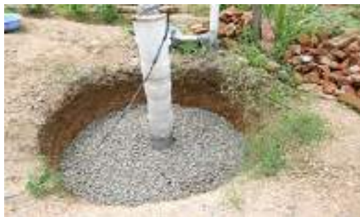
Second layer of angular gravels
