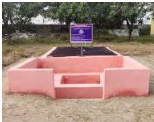
Fig. 1. Groundwater recharge cum drainage unit installed in university campus
