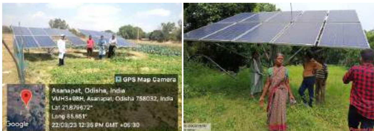
Solar irrigation under PM-KUSUM scheme at Poipani, Odisha
