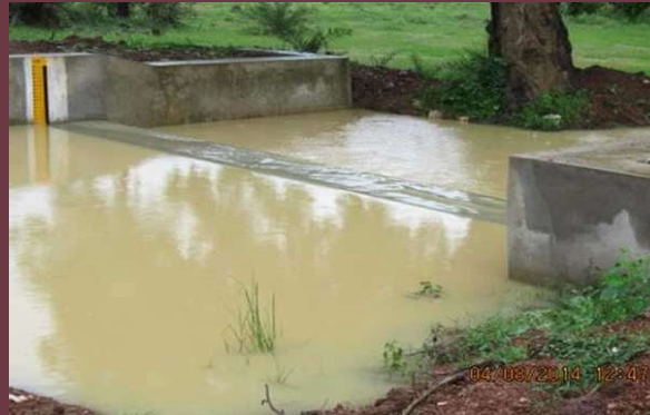
Constructed surplus escape
